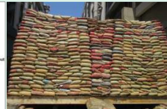
Pile Load Test on Jet Grout Pile
